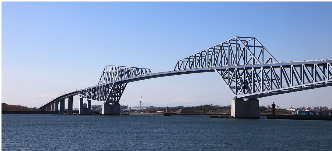
Fig. 1.2-3 Tokyo Gate Bridge with application of SBH500 steel grade to the full-welded truss girder
