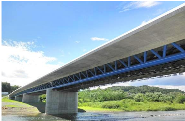
Fig. 1.2-2 Nagata Bridge with application of SBH500 steel grade to the space truss system
