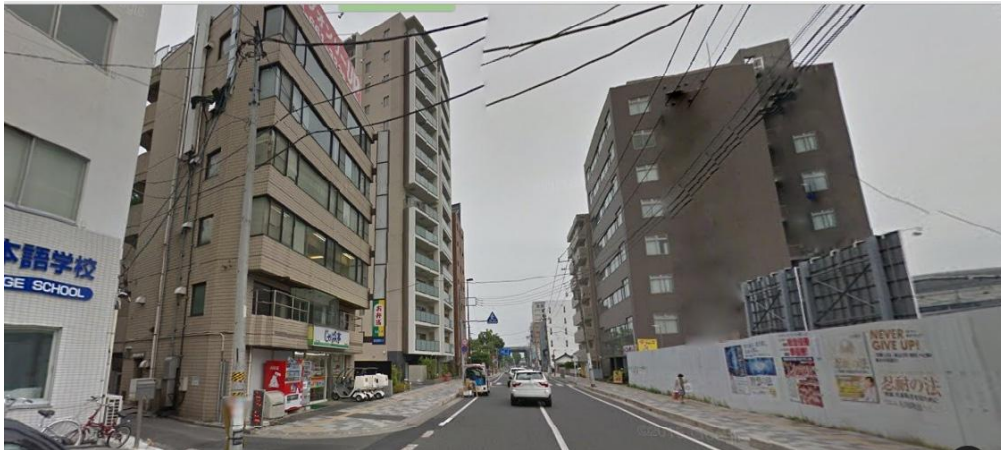
(a) Make Building Appearance Simple by Removing Some Visual Elements
