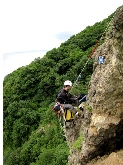
Fig.1 Steep slope operation by rope
