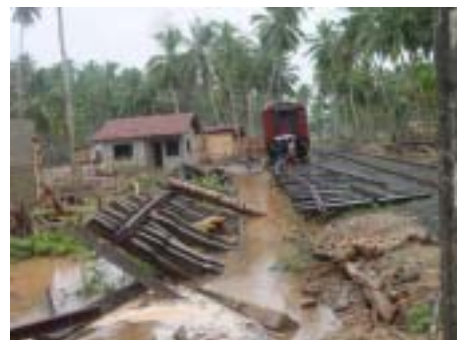
Fig.3 Damaged train and rails at Hikkaduwa
