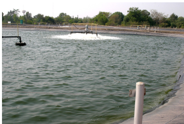
Fig. 13 Aeration lagoon of wastewater treatment plant in Ubon Ratchathani University.
