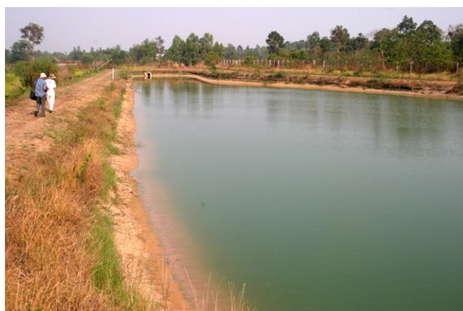
Fig. 15 Final sedimentation pond of wastewater treatment plant in Ubon Ratchathani University.
