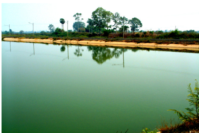
Fig. 10 Third lagoon of Warinchamrap wastewater treatment plant covered with thick Water Bloom.
