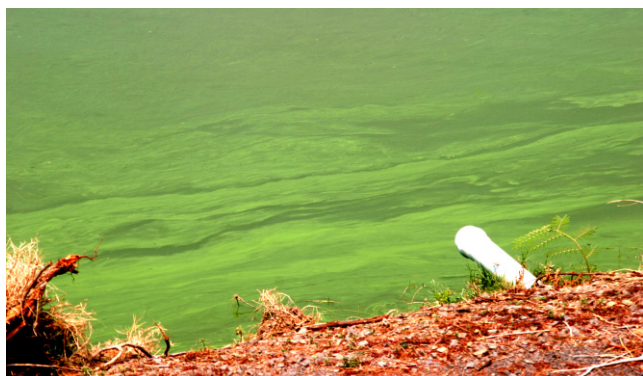
Fig. 12 Second lagoon of Ubon wastewater treatment plant covered with thick Water Bloom.
