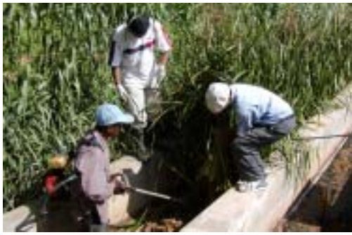
Fig. 1 Constructed wetlands in University of Peradeniya : harvesting of Scirpus grossus .
