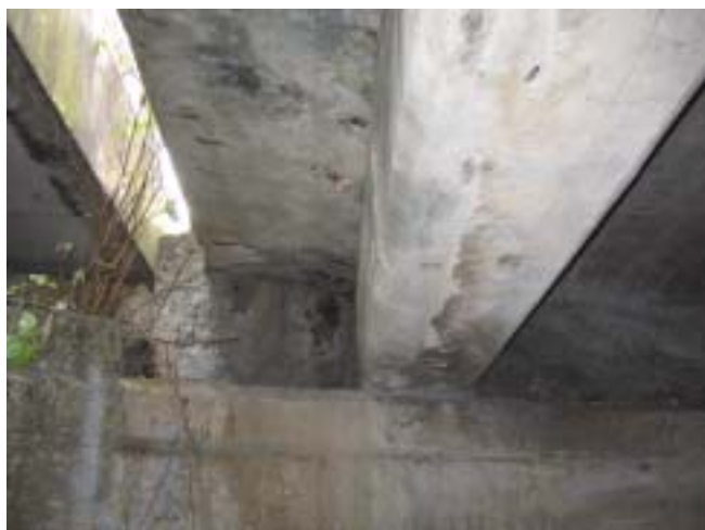
Fig. 3 Condition of main girder and (Bridge A)
