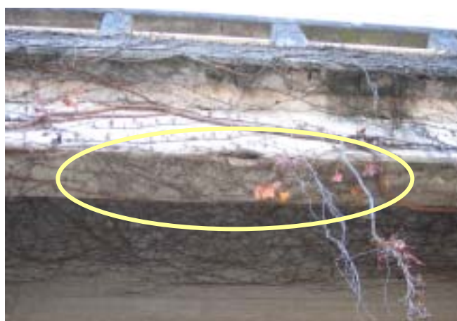
Fig. 6 Condition of main girder (Bridge B)
