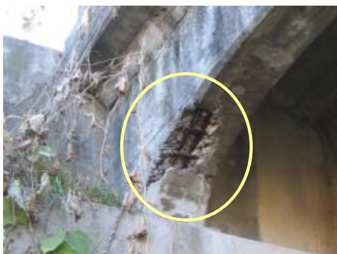
Fig. 5 Condition of main girder near the abutment (Bridge B)
