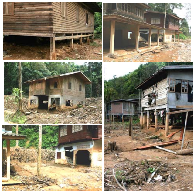
Fig. 13 Remainder houses, Ban Yok Radab
