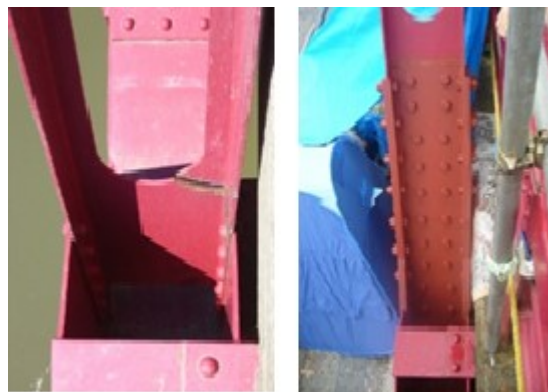
Fig. 5.2. Damaged and reinforced conditions of D5u diagonal member
