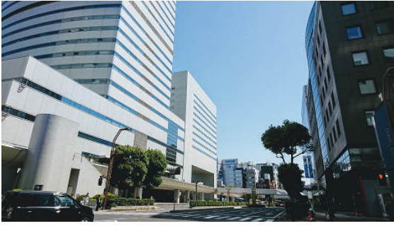
Fig. 2. Photograph of Omiya station's western entrance.
