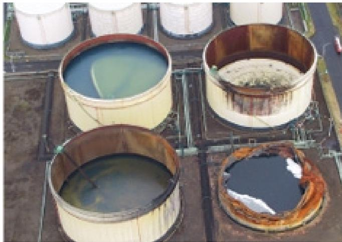
**Fig. 1-1:** Floating roofs sunk during Tokachi-oki earthquake
