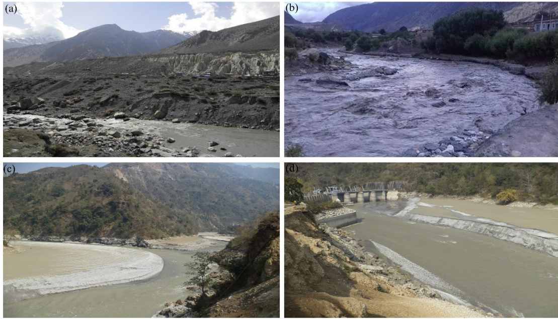
Figure 31. (a) Sources of sediment (b) Sediment transport by fluvial discharge (c) Deposited sediment in KG hydropower reservoir (d) Flushing of deposited sediment in KG hydropower reservoir.
