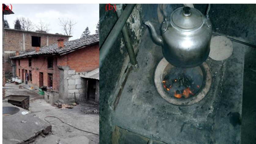
Fig. 5. The stove (a) and building structure (b) in rural Xuanwei, China.
