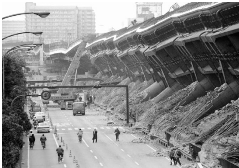
Fig. 1 Fukake Bridge Collapsed due to 1995 Kobe Earthquake
